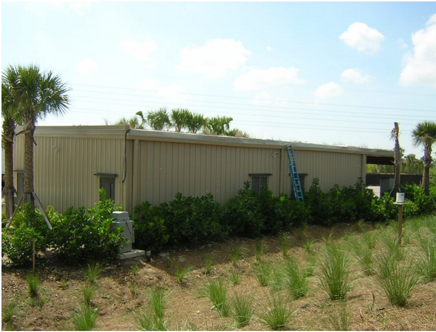
Figure 1-Green Roof Bldg (Golf Course Maintenance Storage) at Shadow Wood Preserve
